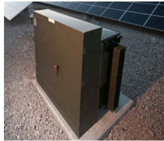
Medium voltage step-up transformer
